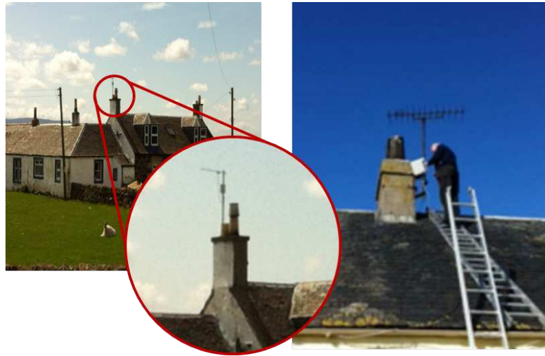
Figure 9.3: CPE installations at trialists' premises.
