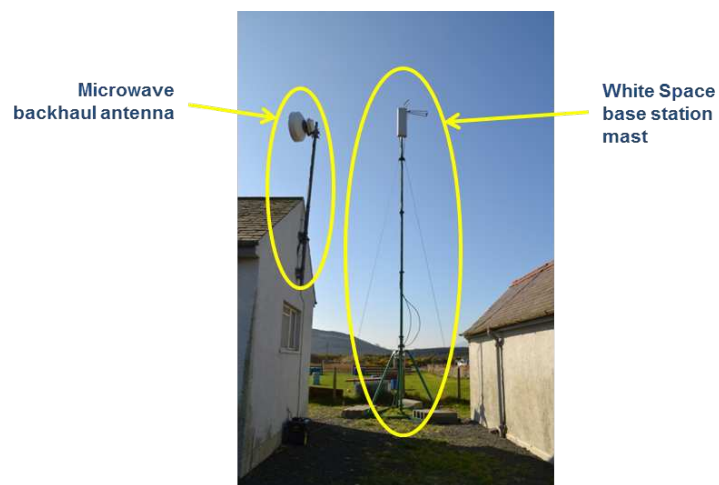
Figure 9.4: White space base station mast at local telephone exchange. (The 18 GHz backhaul dish antenna is also visible.)
