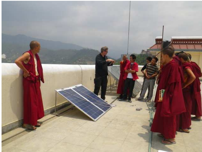
Figure 13.3: Powering teachers' computer room at the Kopan monastery school, Nepal.
